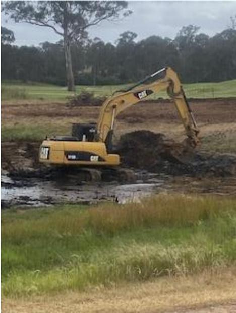
The dam on the side of the 18<sup>th</sup> tees was de silted, filled in, compacted and then the new tees were shaped onto the area
