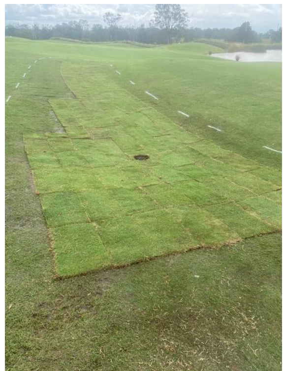
FINISHED PRODUCT AFTER GRAVEL AND SAND IS PLACED IN TRENCH
