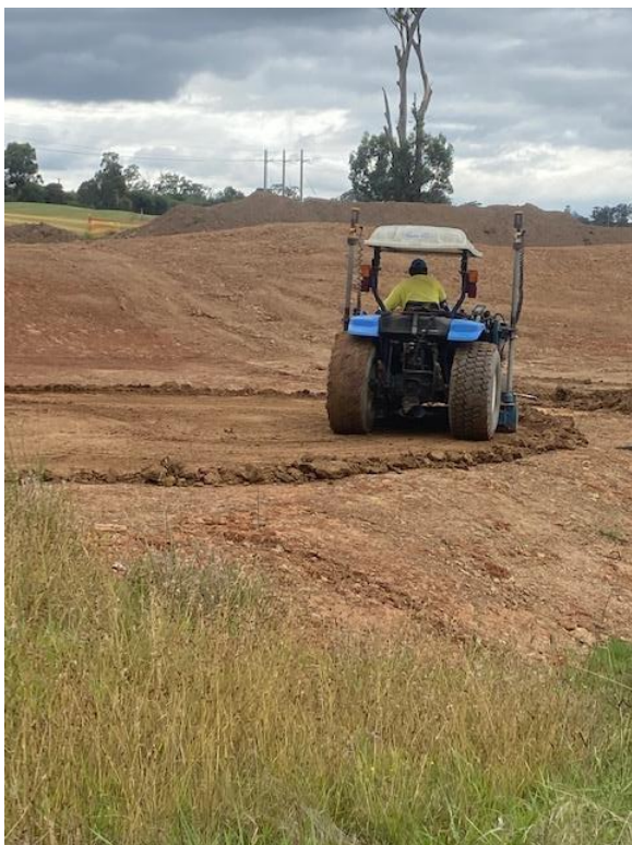
Laser levelling of tee platforms
