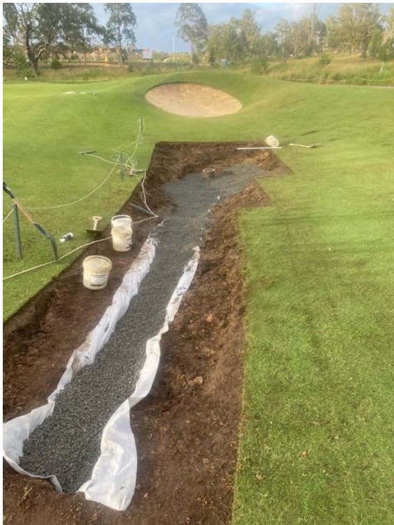
FINISHED PRODUCT AFTER GRAVEL AND SAND IS PLACED IN TRENCH
