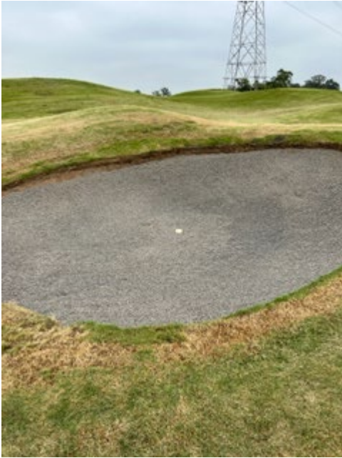
LHS – Drainage 10mm gravel covers the whole bunker RHS- Finished with sand covering the gravel
