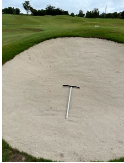
LHS – Drainage 10mm gravel covers the whole bunker RHS- Finished with sand covering the gravel
