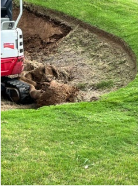
15 th Fairway Bunkers LHS- Stripping of the bunker RHS- Drainage line dug out and old drainage outlet flushed
