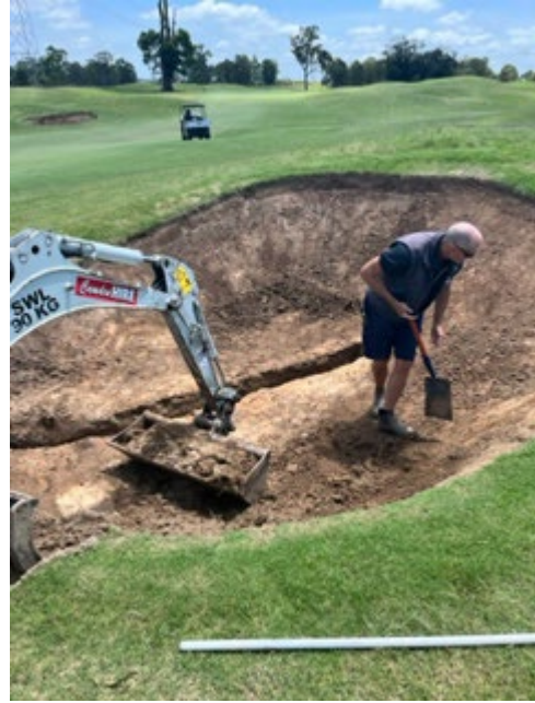
15 th Fairway Bunkers LHS- Stripping of the bunker RHS- Drainage line dug out and old drainage outlet flushed
