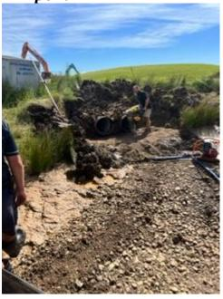
A drop box structure was installed after a change to engineer's drawings for the discharge of water from this dam. This meant an increase in height of water for this water feature. A much better outcome for the course.
