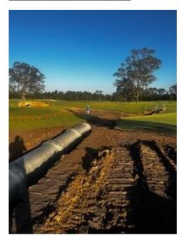
On the RHS golfers would notice the wet area from the development and the need to send all traffic between the basins. This is now getting a solution put in place that will also see a 750mm stormwater pipe installed and over this will be access for our cart path.
